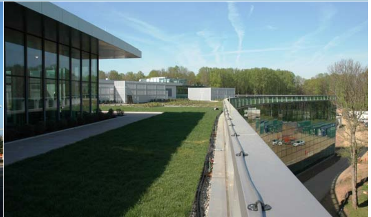
SAP America's second corporate headquarters in Newtown Square was designed to LEED Platinum standards, with numerous sustainable design features including a green roof (pictured), a floor-to-ceiling glass exterior to take advantage of natural daylight, a rainwater cistern, and geothermal heating and cooling. Photo © SAP AG 2009. All rights reserved.
